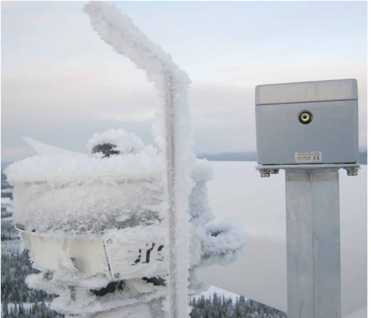
Light sensor unit (heated) on top of the nacelle
